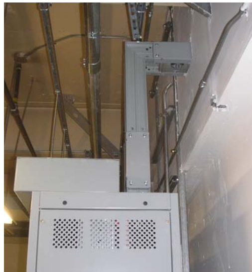
Side view of the transition to 1,200 A busway
